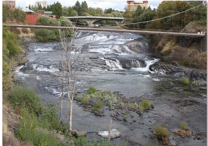
The North Channel of the Spokane River after Avista constructed weirs (small dams) in the river channel which were so cleverly designed that the approximately 170 cfs flowing in the river in this photo has the same appearance as 1500-1600 cfs did prior to the project completion. These weirs are indistinguishable to the public, as they were color and texture matched to blend in with the surrounding basalt channel.
