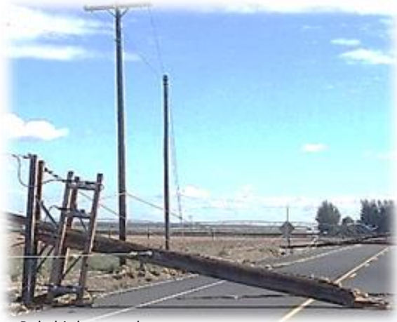
Pole hit by a truck
