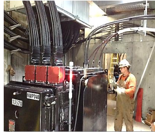
Downtown Network Vault
