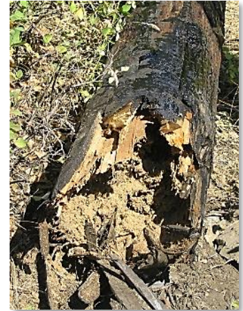
Pole rot causes a failure
