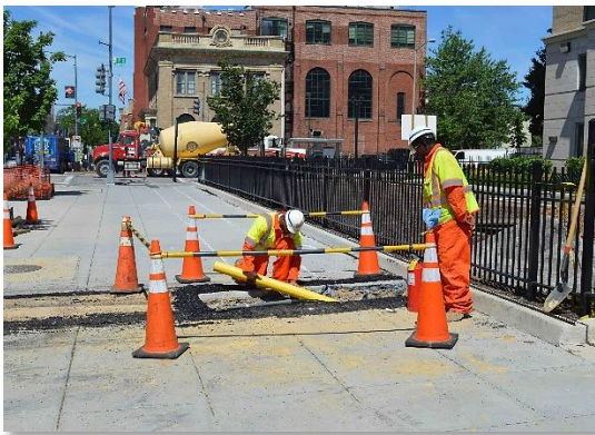
Natural Gas Pipeline Repair in Downtown Spokane
